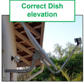
Figure 7 - Incorrect and correct offset dish elevation (applicate for Namibia and South Africa)
